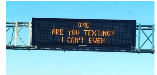
Figure 10. Example of electronic signage (Source: Illinois DOT, https://newschannel20.com/news/local/unusual-highway-signs-grab-drivers-attention )
