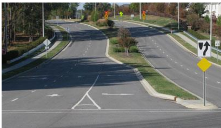
Figure 4: Example of a Raised Median
