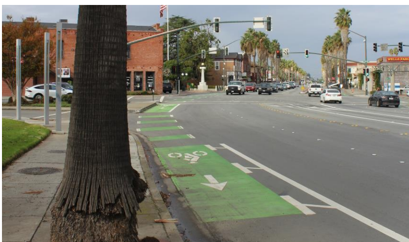
Figure 33: Example of Bike Lane Extension Through Intersection
