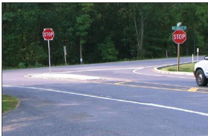
Figure 24: Example of Splitter Island
