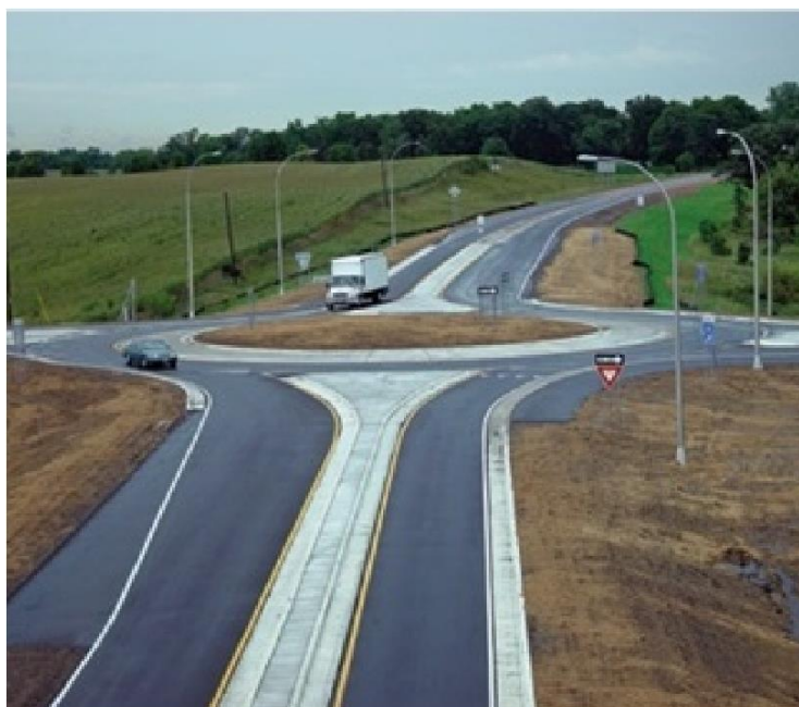
Figure 13: Example of Single Lane Roundabout
