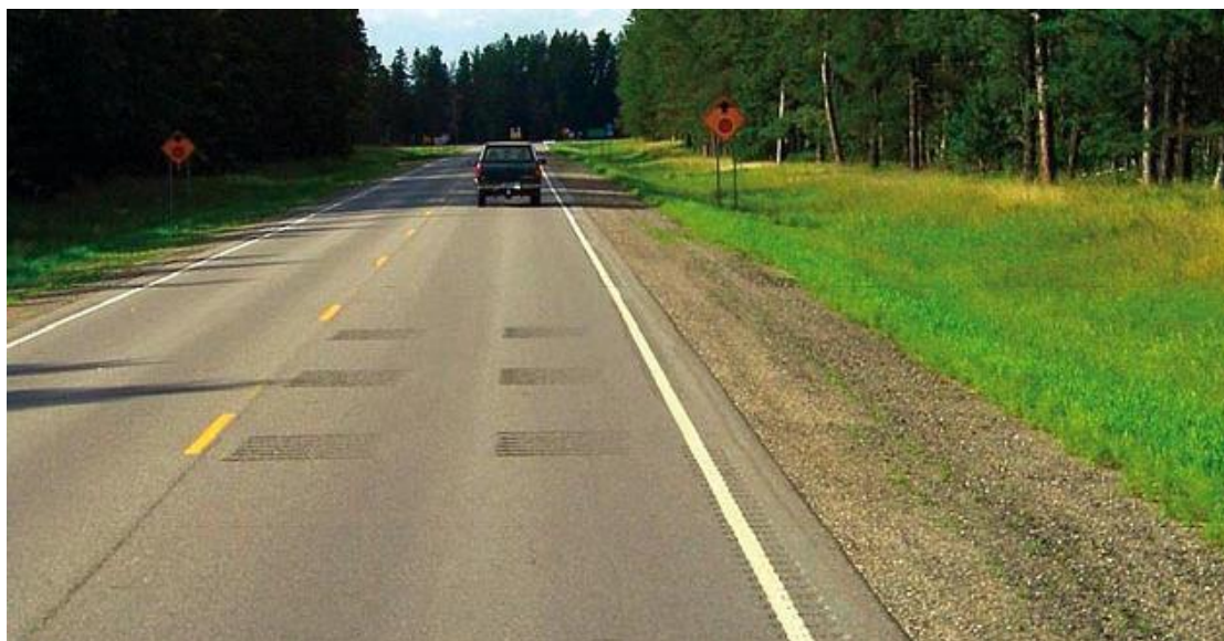
Figure 16: Example of Transverse Rumble Strips
