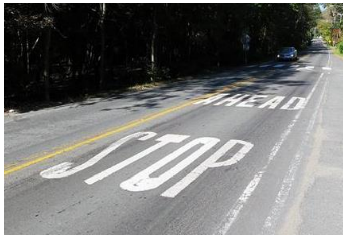
Figure 23: Example Pavement Markings at an Intersection
