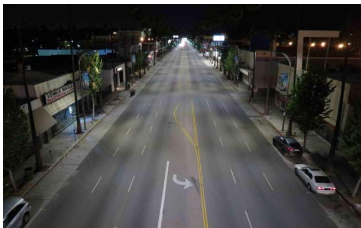
Figure 1: Example Lighting on the Roadway
