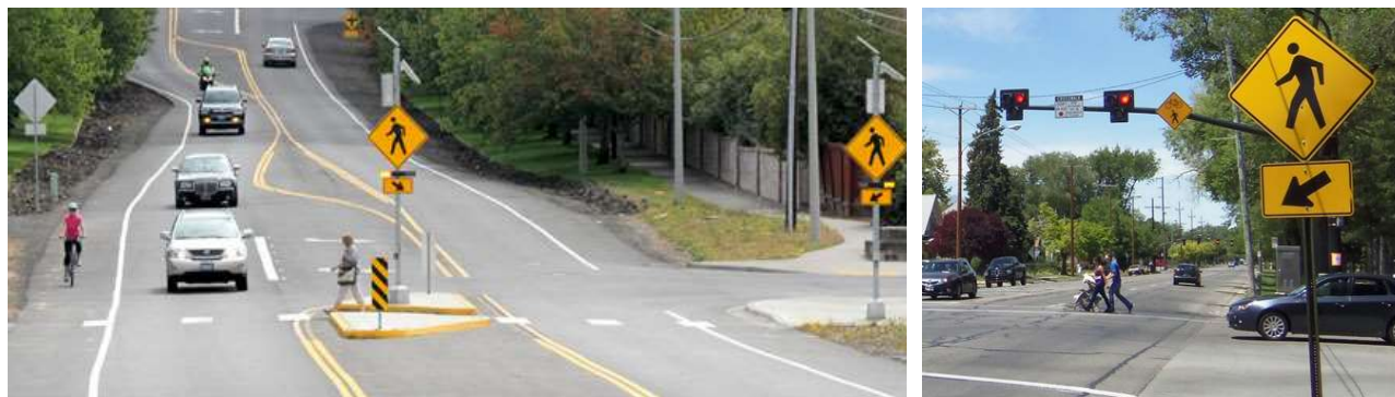
Figure 31: Example of Enhanced Pedestrian Crossing
