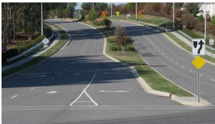
Figure 4: Example of a Raised Median
