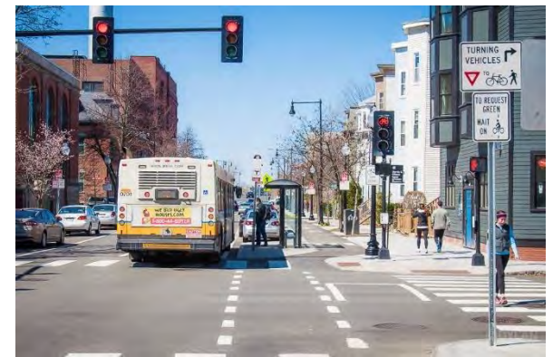
Figure 26: A concrete curb-separated bike lane (top); bike lane bending out to traverse behind transit boarding island (bottom).
