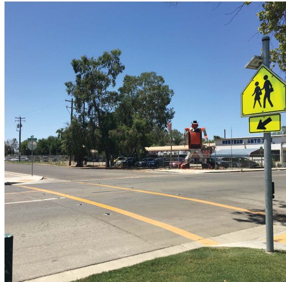
Crosswalk with in-pavement flashers in the unincorporated community of Riverdale.
