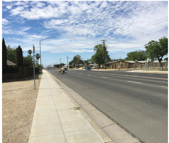
Pedestrian crosses Derrick Avenue (SR 33) at unmarked location in Mendota.
